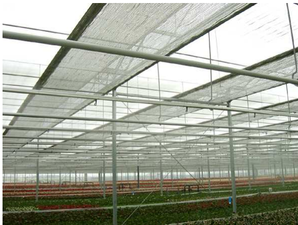
Moveable screen for optimum light level
